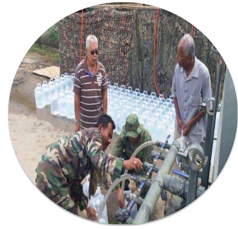
Require electricity & pumps
